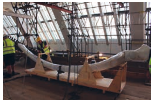
Figure 7. Each mandible was carefully packed into a bespoke wooden cradle and then lowered to the ground.
