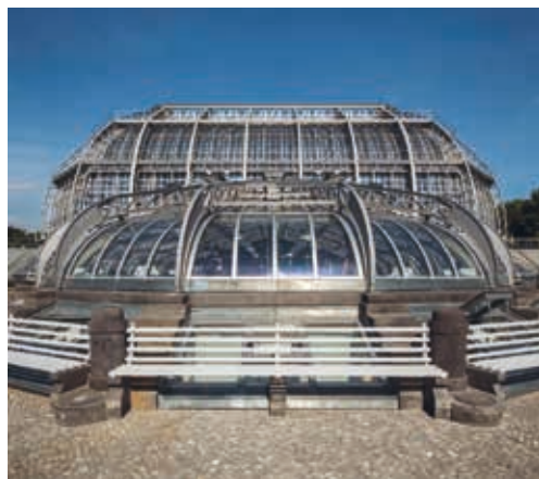
Figure 1. Large Tropical Conservatory after the renovation, Victoria House in the front (Photo: Dirk Altenkirch).
