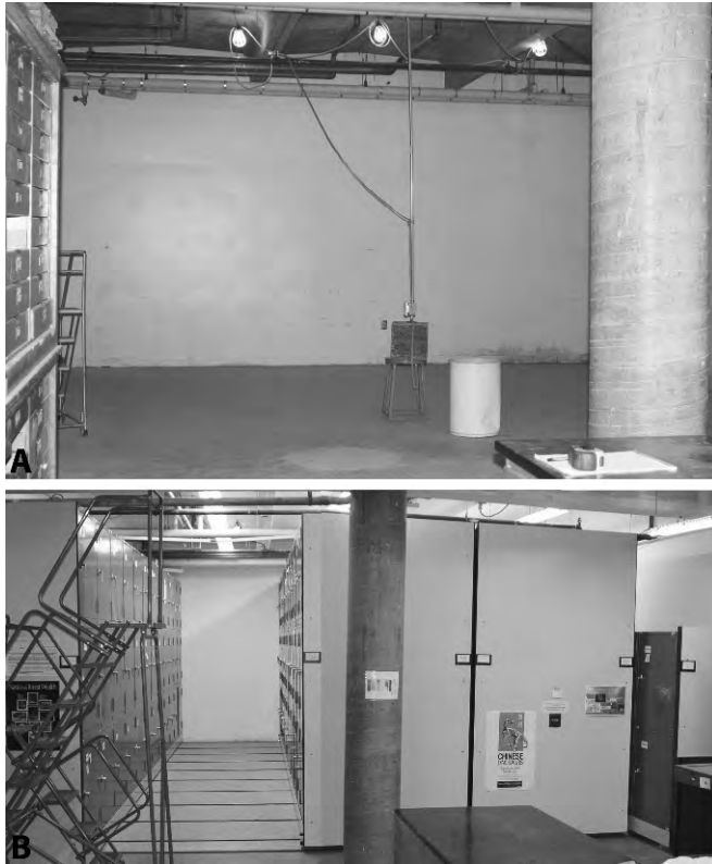
Figure 2. (A) The University of Montana Paleontology Center (UMPC) collection room during the renovation. (B) After the renovation (repainting, new lighting) with the compactor system installed.
