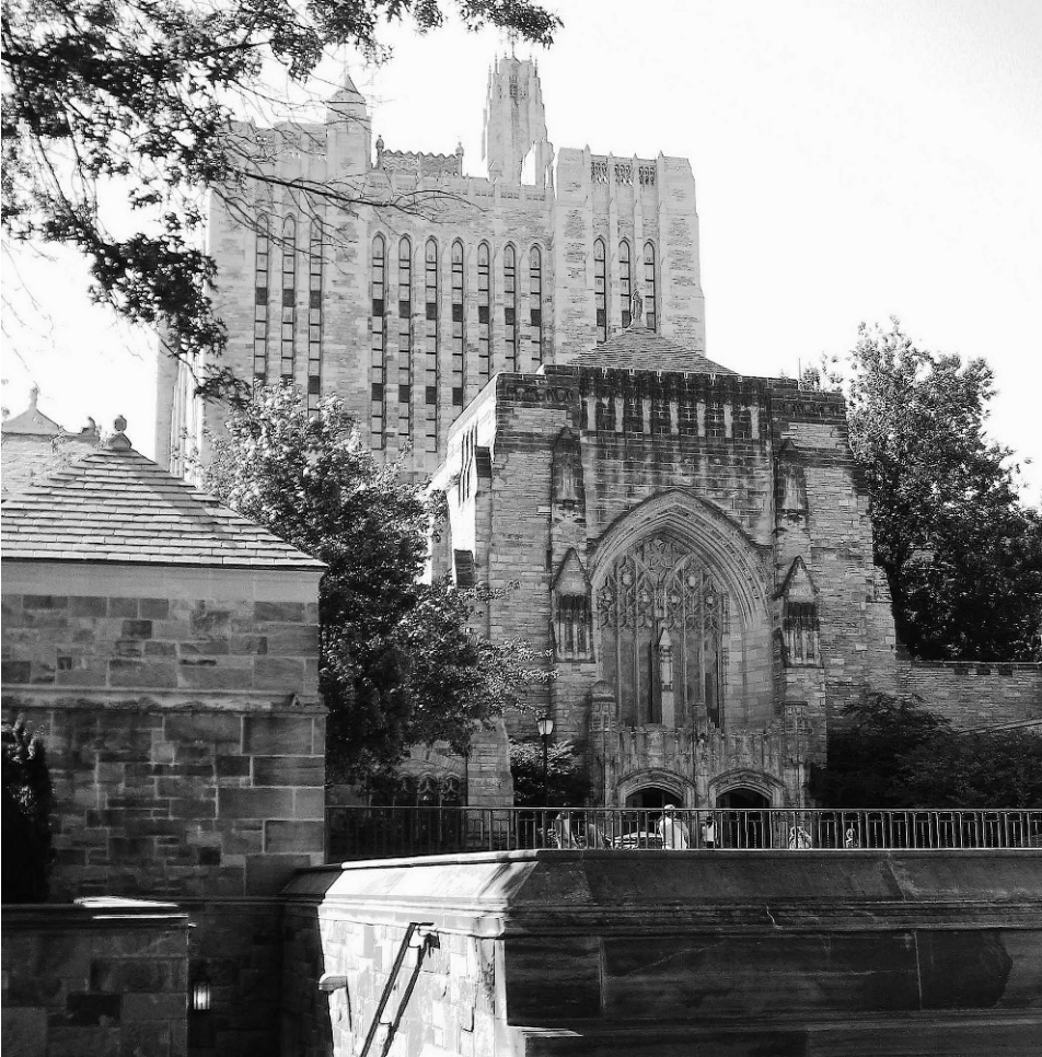
Figure 1. Yale University's Sterling Memorial Library includes 14 stack levels served by six different air-handling units. The shutdown experiment involves turning off all six units for 8 hours each night.
