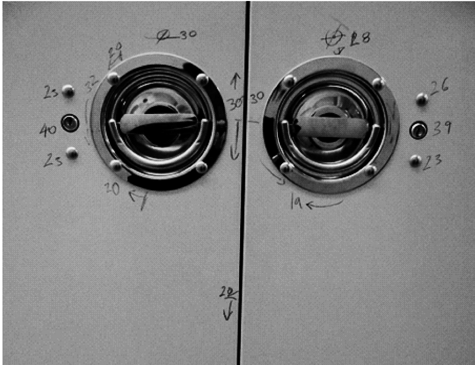
Figure 2. Cabinets marked after testing with an ultrasonic leak detector, which records “leaks” as dBmV readings of sound escaping from various parts of the cabinet. The sound was produced by an ultrasonic emitter placed in each cabinet. Readings were recorded directly on the cabinets using a wax pencil.
